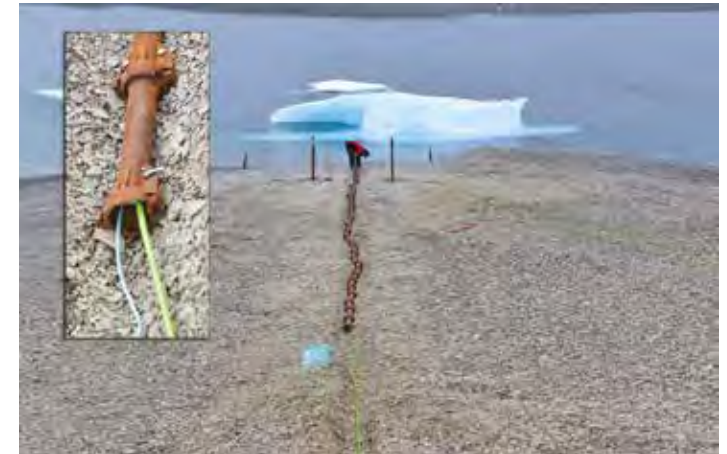
Figure 3 - Articulated pipe being installed for an Arctic test to protect subsea ethernet cable. A diver-free installation method was used and has so far protected the cable from potentially damaging ice conditions. (Image courtesy of Ocean Networks Canada)
